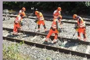
Off Track Tamping
