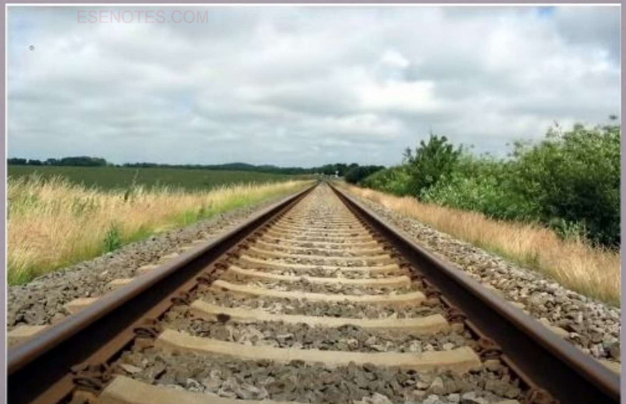
Adzing of Sleepers
