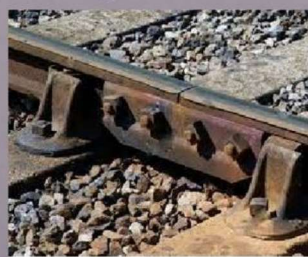
Bridge Joint with Metal Flat
