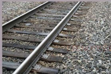
Broken Stone Ballast
