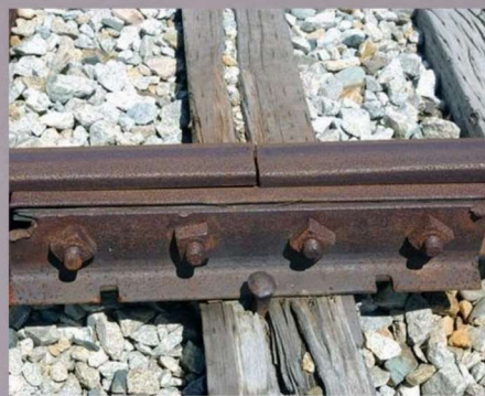
Supported Rail Joint
